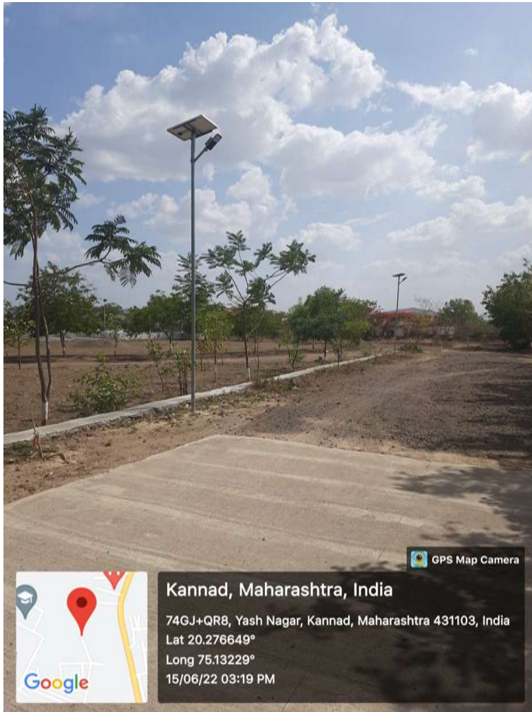
1.Solar Energy LED Street Light
