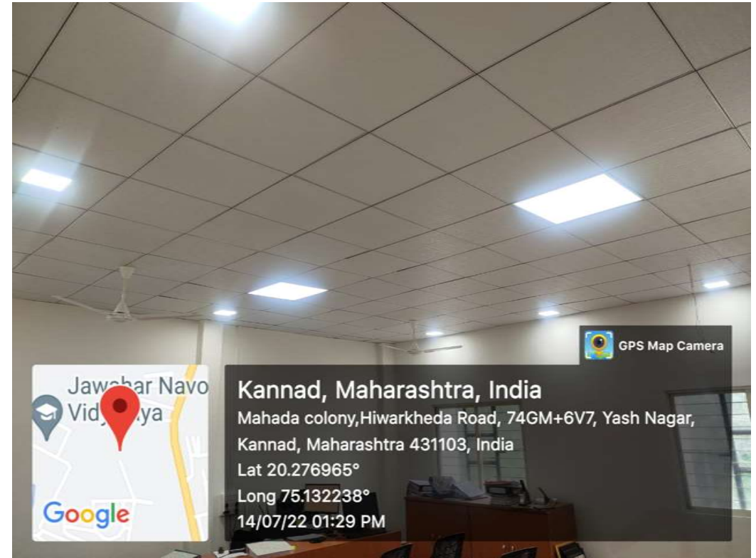
16. LED Lights in Office
